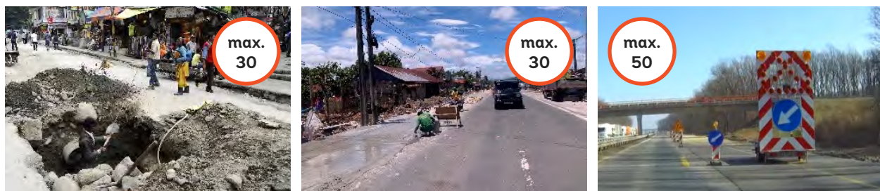
Figure 13. Typical examples of roadwork zones
