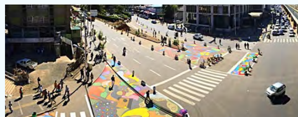
Addis Ababa – Tactical urbanism before (above) and after (below) showing the painted curb and median extensions, crosswalks and lane markings added to narrow the road and prioritize pedestrian safety
